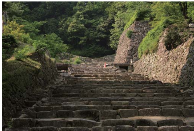
Otemichi road following restoration
